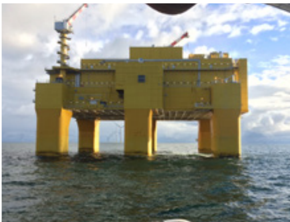
Power station for a wind farm in the North Sea
